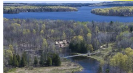
Hodenpyl Pond and suspension bridge
